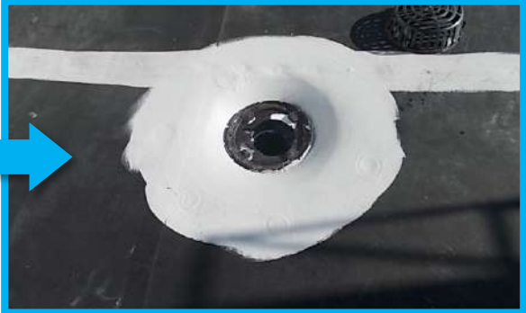
Seal and waterproof drains
