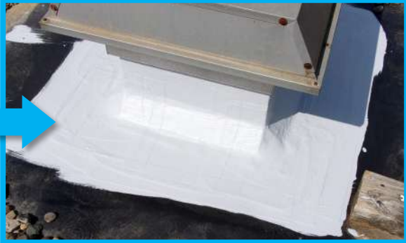
Seal and waterproof penetrations
