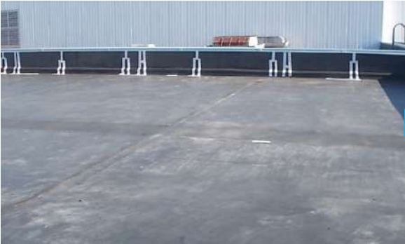
Deeply embedded particles
