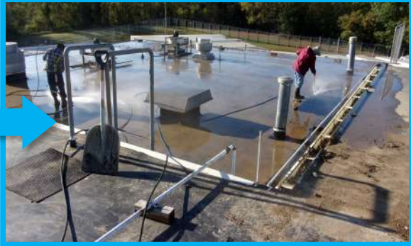
Pressure wash and clean entire roof
