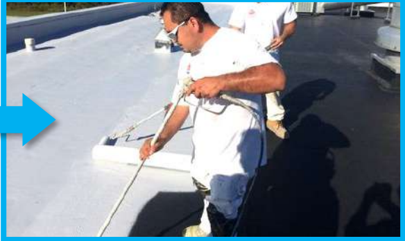
Fully-reinforce entire roof creating monolithic system
