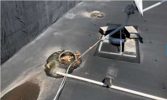
Failing drains
