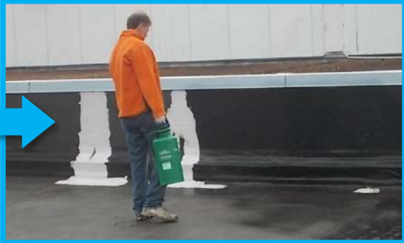
Treat roof with ASTEC Rinseable Primer, removing chalkiness
