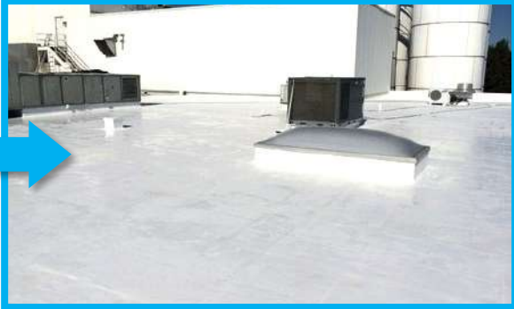
Fully-reinforced ASTEC System minimum 50 mils (DFT)
