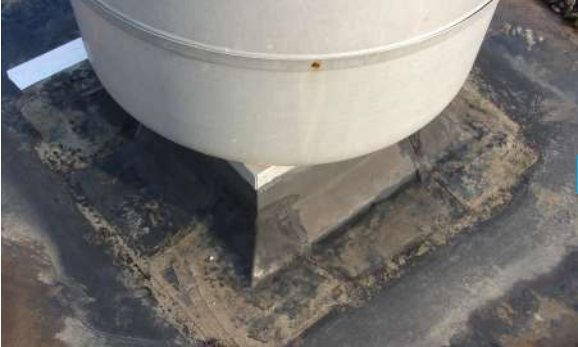
Failing penetrations
