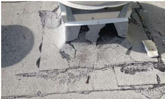
Failing penetrations
