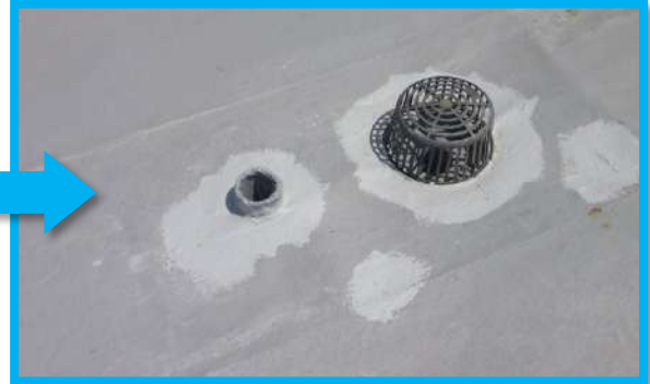
Seal and waterproof drains
