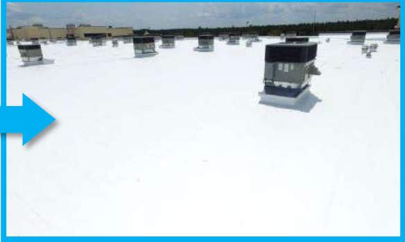
Fully-reinforced ASTEC System minimum 50 mils (DFT)
