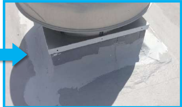
Seal and waterproof penetrations
