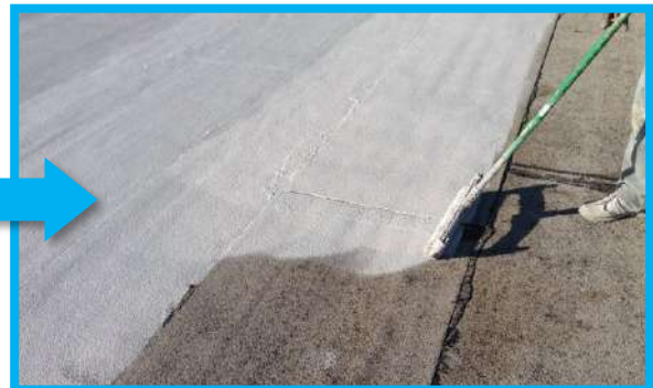
Sealing the substrate
