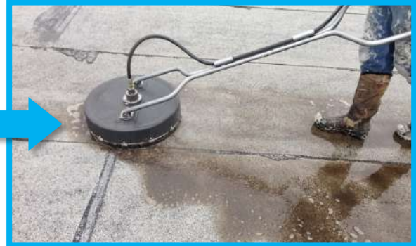
Remove debris and thoroughly clean the entire roof
