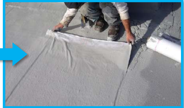
Fully-reinforce entire roof creating monolithic system
