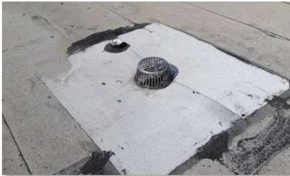
Failing drains
