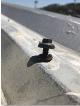
Fasteners backing out and dirt and debris buildup
