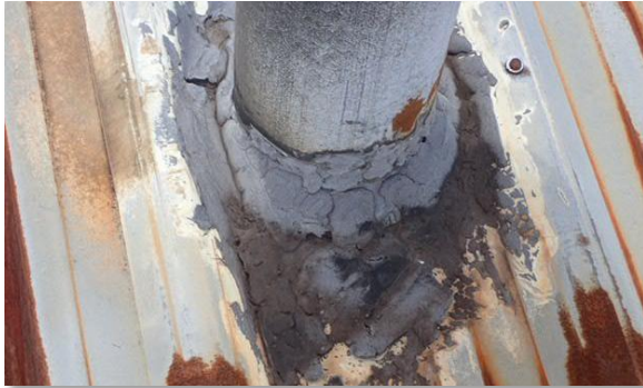
Failing penetrations
