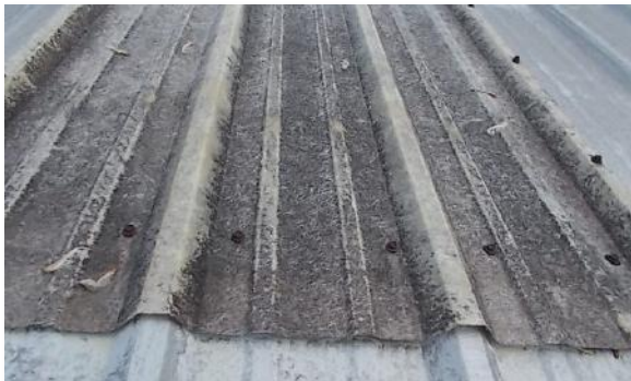
Deteriorating skylights
